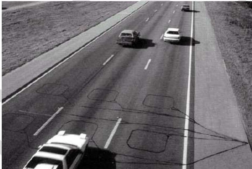
Figure 5. Double loop detectors in practice
