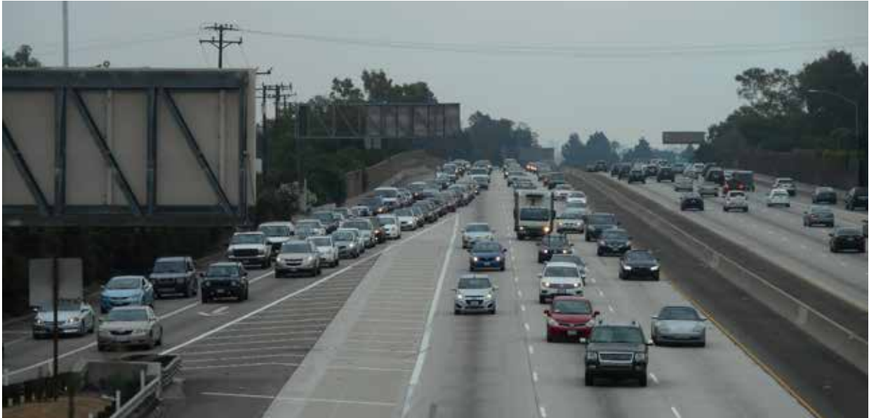
I-10 OFF-RAMP AT CLOVERFIELD BLVD
