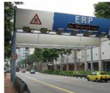
Full Span Gantry (Singapore)
